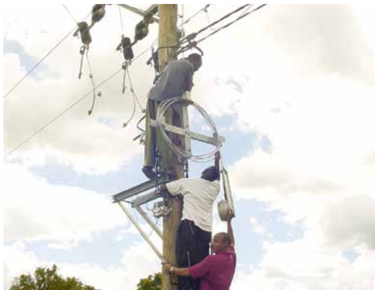
Installation of solar-powered router in Tanzania.
